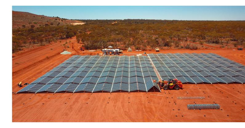
5B Maverick layout. Within a 5B Maverick layout, Mavericks that have their long sides exposed to the wind are classified as 'External' while those that are within the array and shielded from the wind are classified as 'Internal' Combinations of different Internal and External 5B Maverick models provide for cost effective layout for a given load condition.
